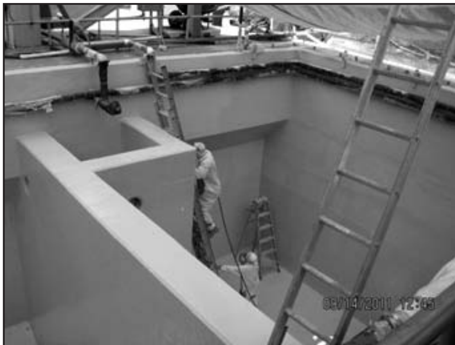
Rehabilitation of the new sludge storage tank. Note: new dividing was in the foreground.
