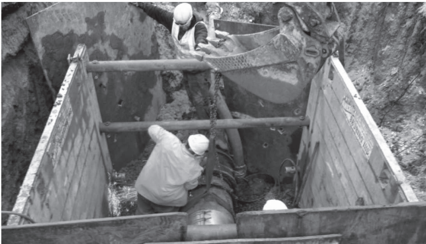
Final adjustments to complete the sewer main repair
