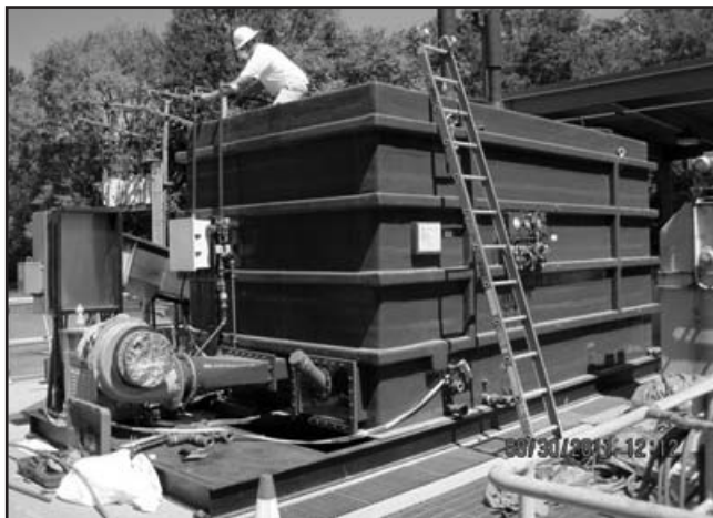
New Biofilter/Biotrickling Filter Installation
